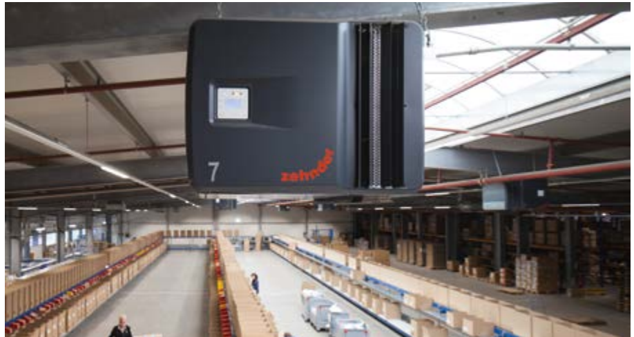
High dust levels in the logistics facilities resulted in contaminated goods at NTL. Despite expensive cleaning procedures, customer complaints repeatedly occurred. With the help of industrial air cleaning, this problem could be managed successfully.
