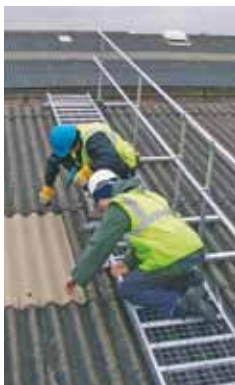
Short duration maintenance
