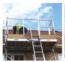
**Winged Gates:** Provide additional edge protection over and above that of the standard 2m wide Easi-Dec Platform. Tested to EN13374 Class C.
