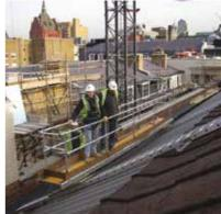
Designed for use on industrial and fragile roofs, Roof-Walk is a fully guarded rolling work platform mounted on twin tracks to enable movement up and down the roof. Roof-Walk's rolling platform is available as standard 4.6m or it can be specially made as a 2.5m platform if required. The system runs up and down twin modular 4m linking track sections which are fitted with safety mesh and support battens.
