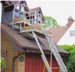
**Double Dorma Kit:** Allows additional platforms to be positioned up to the roof. With a platform and Dormer Kit already in position, the next platform is fitted with a pair of padded 'dormer bars' and telescopic struts to comprise a Double Dormer Kit. Safety note: All Double Dormer Kits must be attached to the building.
